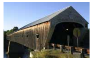
Cornish Windsor Bridge Two
