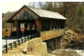
Packard Hill Bridge
